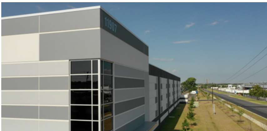
Geneva II Warehouse in Charlotte, NC.
