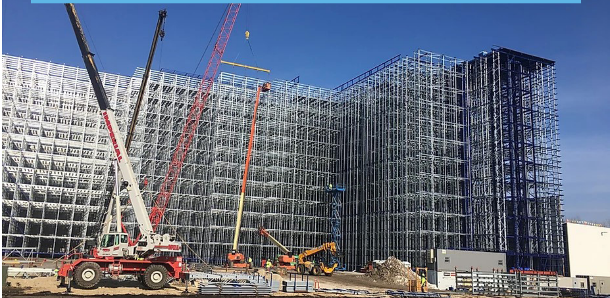
The 130-foot-tall Americold Automated Storage and Retrieval System under construction in Rochelle, Illinois (above) and completed (below). Photos courtesy of Griffco Design/Build, Inc.
